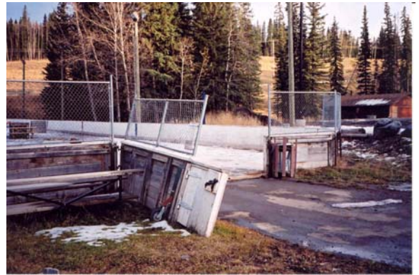
Calgary Area Rink Photo Courtesy of GWS Technologies Ltd
